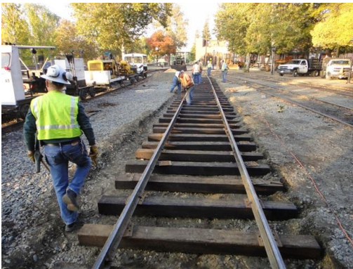
The ties are down, the rail is in place and now John R., Heather, Steve, Clem, and Ed in the foreground put in the joint bars.
