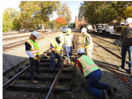
Roger, Frank, Steve, John, Mike are placing the tie plates, pre drilling and spiking the rail while DRO Hardy stands in awe of the MOW crew skill.
