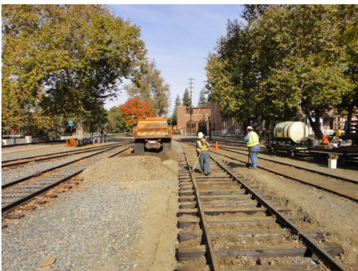
Putting in the ballast! Heather and Frank work the shovels while the truck delivers more rock.
