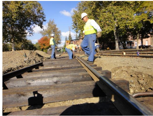
The ties are in and now Clem, Ed, and Mike move the vintage 1887 rail back into place on the new ties.
