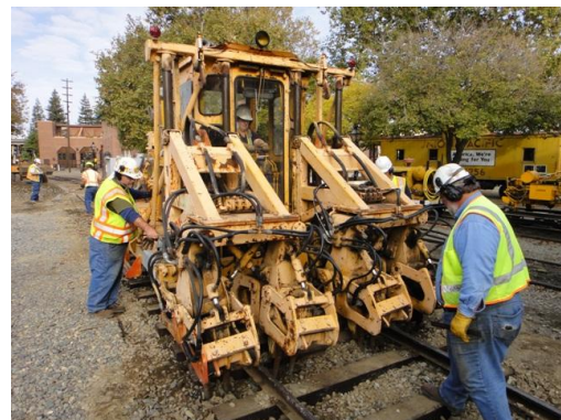
Heather runs the tamper under Frank's direction while Mike monitors from the side.
